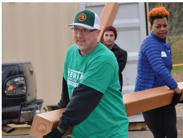
Dr. Thomas Huebner lends a helping hand at the construction site.
